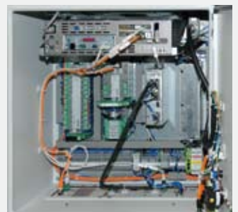
EPS electric pneumatic installation system with embedded system micro controller and electrical interfaces to PLC
